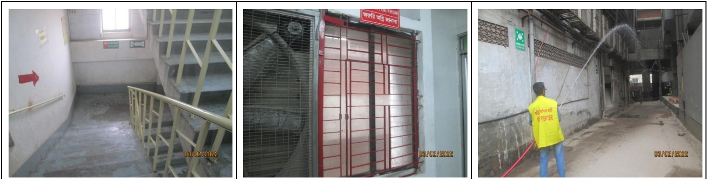
Staircase Bare window Fire hose check by fire fighter
