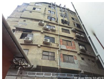
Facility Building View.jpg
