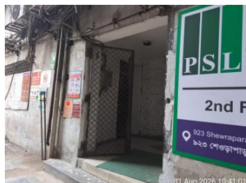
Facility Main Gate View.jpg
